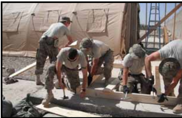
Above: 577 EPBG Airmen framing walls for the much anticipated Dining Facility at FOB Kunduz. The aggressive construction schedule on this project enabled the 2-18 IN BN to enjoy a LOGCAP prepared Christmas meal. Merry Christmas Army – from the Air Force!
