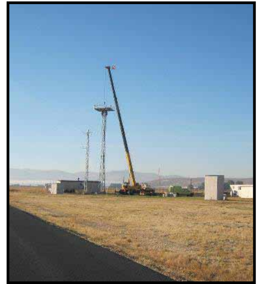
A tower is erected near the trap and skeet range on the south end of Kingsley Field. Three towers like this one have been installed at the base and ensure enhanced radio communications now and in the future. (Photo by Chief Master Sgt. Todd Berndt, 173rd Communications Flight.)
