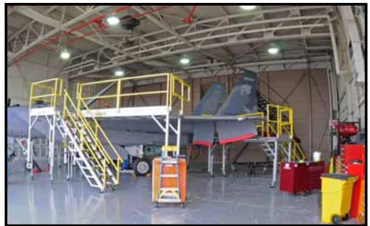
Bld. 400 houses jets in phase maintenance following some renovations to the historic buildings. The stands pictured meet the requirement for passive fall restraint and personnel using them say they speed the phase maintenance process. (U.S. Air National Guard photo by Master Sgt. Jennifer Shirar, 173rd Fighter Wing Public Affairs)
